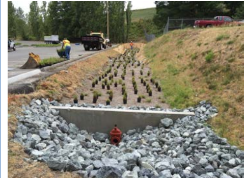
Logistics Bioretention Swale
